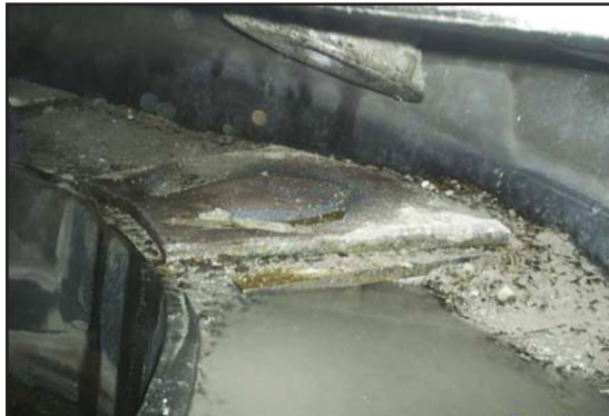
Discharge cone above wear plate
